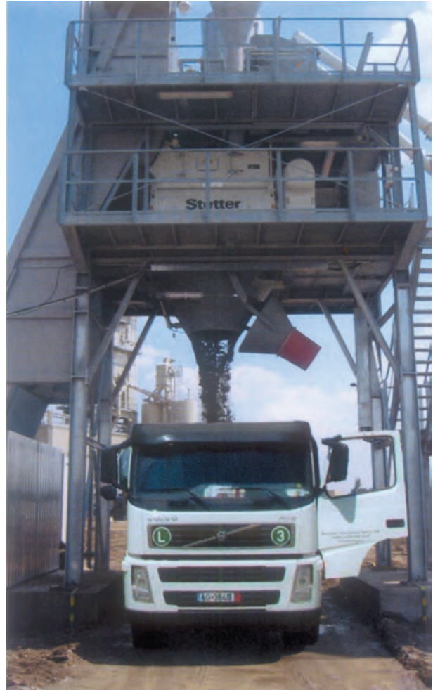
Discharge into open truck.
