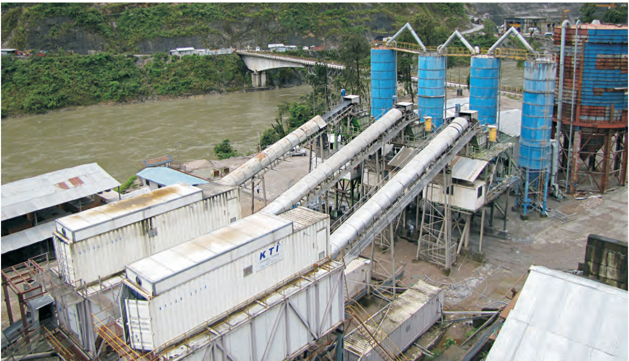
The H6 plant at Subansiri in dam concrete that set record in PQC production (6020 cu.m in 1 day)
